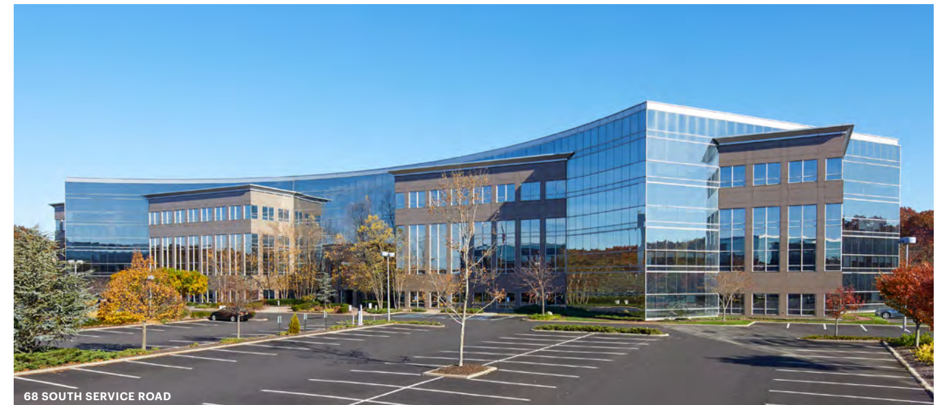
68 SOUTH SERVICE ROAD
